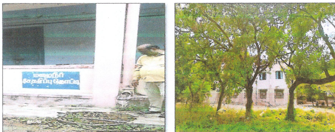
Fig.4. Rain Water Harvesting Pits
